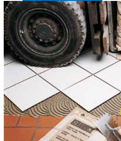
Rapid overlaying on asphalt industrial floor
