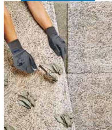
Laying heavy insulation panels
