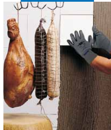
Repair work in a refrigerator unit
