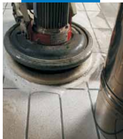
Cleaning off Kerapoxy P with water and a single head rotary machine with Scotch-Brite®
