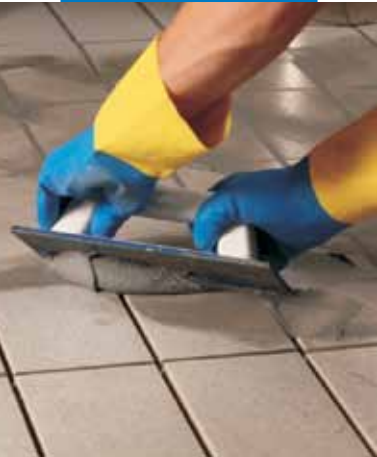
Grouting floor joints with a rubber trowel
