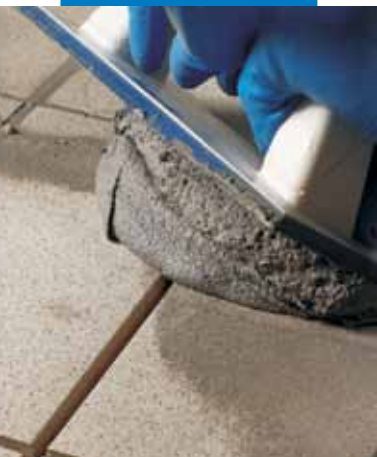
Grouting floor joints with a rubber trowel
