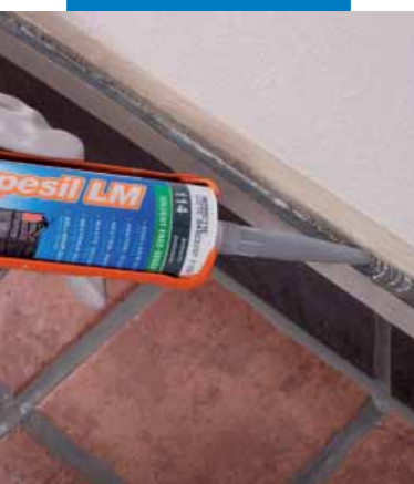
Sealing an internal stone dressing
