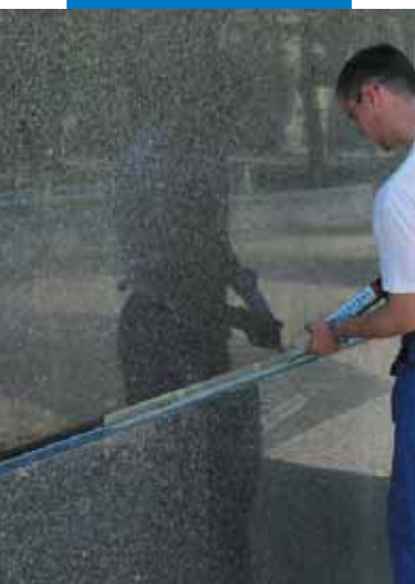
Sealing a façade joint with Mapesil LM
