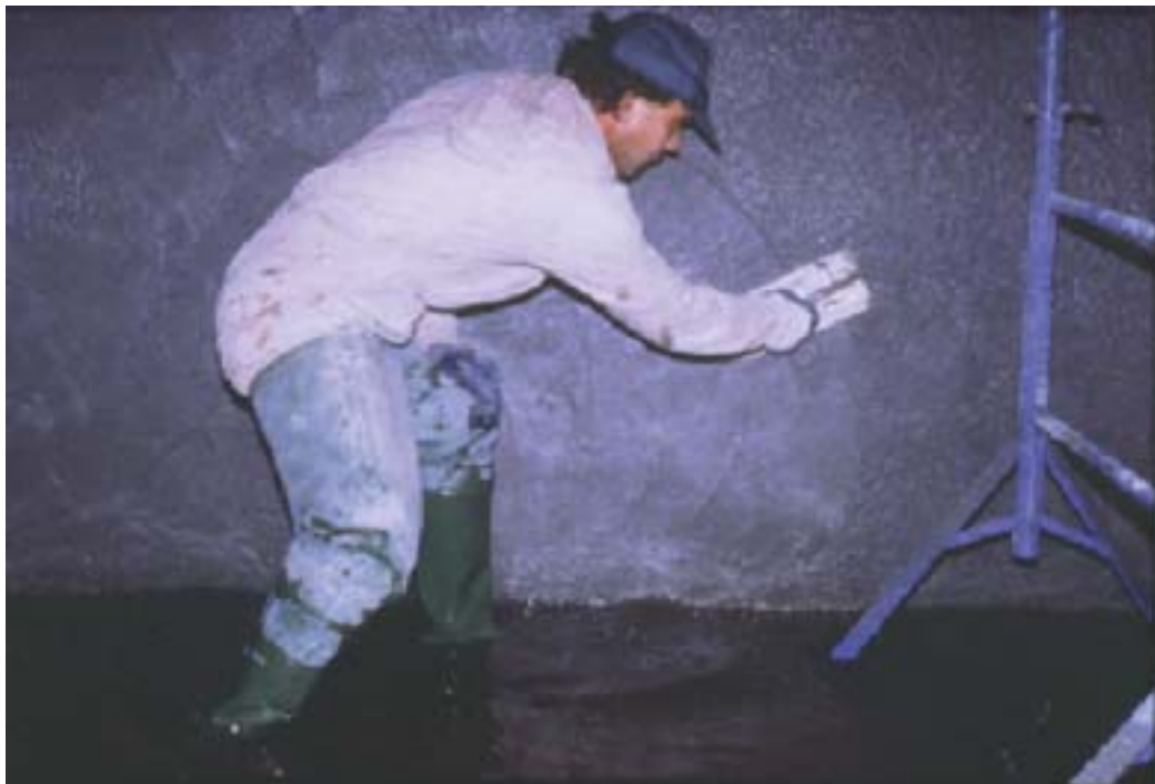
Finishing the surfaces repaired with sprayed Sewament 10
