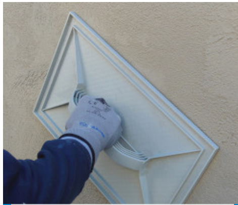
Levelling off the surface of MapeWall Intonaco Base
