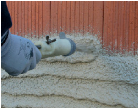
Application of MapeWall Intonaco Base with a rendering machine on a new wall made from perforated bricks
