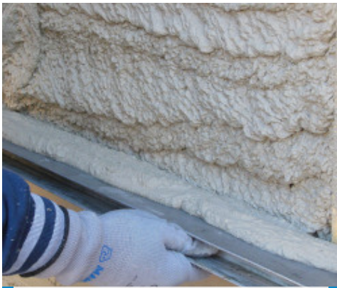
Flattening the surface of MapeWall Intonaco Base with a straight-edge
