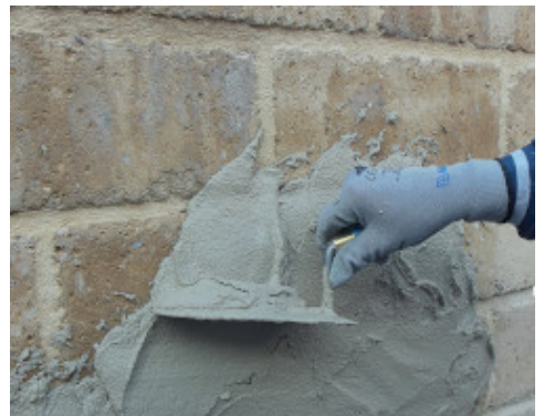
Application of MapeWall Intonaco Base with a trowel on a wall made from blocks of tuff
