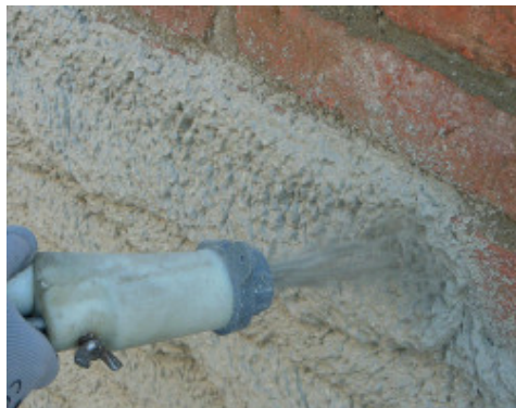
Application of MapeWall Intonaco Base with a rendering machine on a wall made from solid bricks
