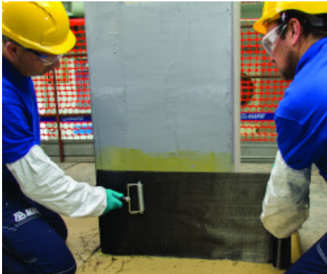
Application of MapeWrap C UNI-AX fibre impregnated with MapeWrap 31
