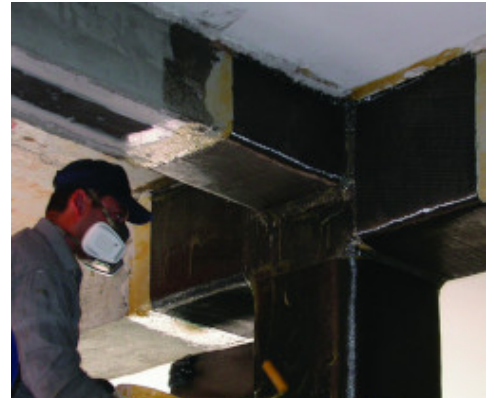
Beam-pillar joints confined with MapeWrap C UNI-AX System
