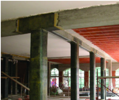
Joints and pillars strengthened with MapeWrap C UNI-AX System
