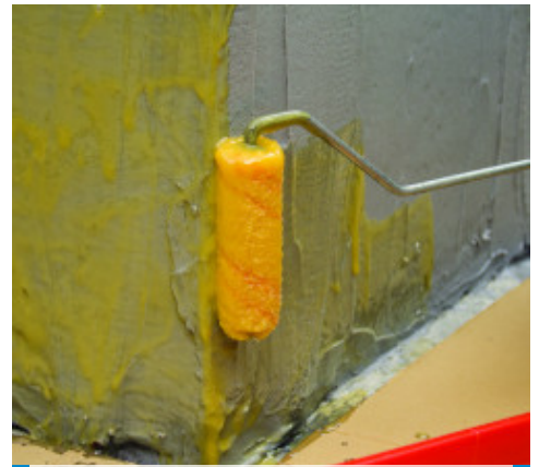
First coat of MapeWrap 31
