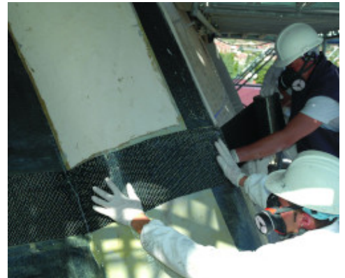
Domed roof strengthened with MapeWrap C UNI-AX System
