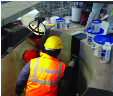
Brickwork chimney strengthened with MapeWrap C UNI-AX System
