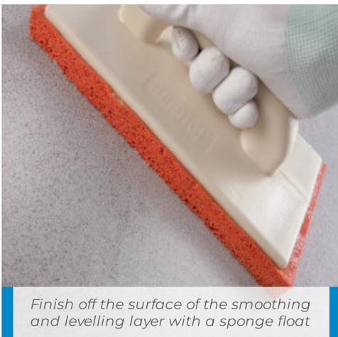
Finish off the surface of the smoothing and levelling layer with a sponge float
