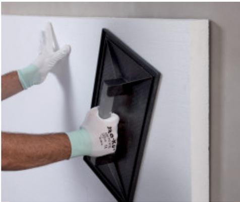
Press the panel in place to guarantee a good bond to the substrate
