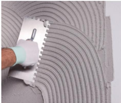
Lay the first coating of smoothing compound with Mapetherm ARI GG
