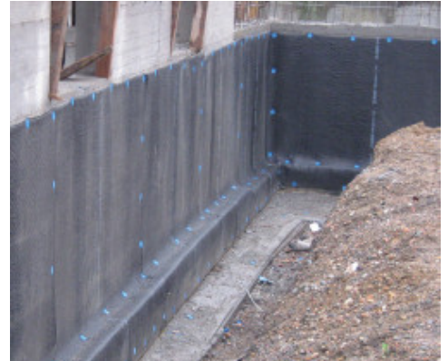
Waterproofing vertical surfaces after pouring
