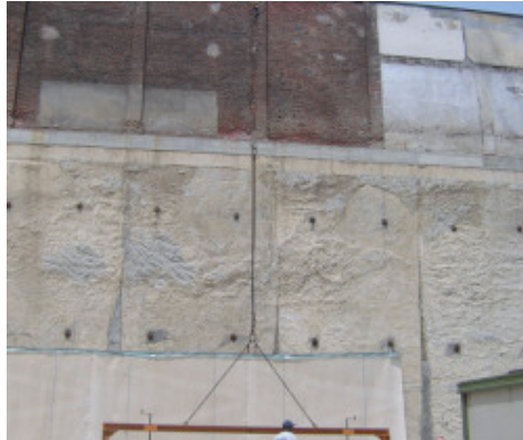
Waterproofing vertical surfaces made up of diaphragms
