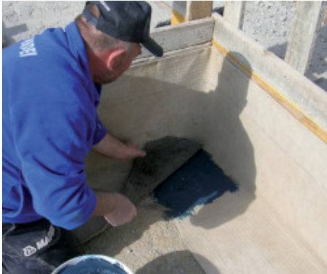
Grouting a corner of the sheet with Mapeproof Mastic
