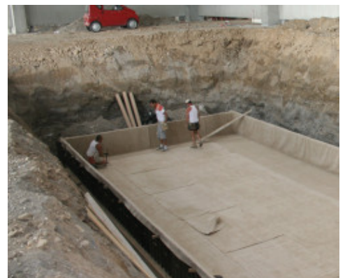
Waterproofing a horizontal surface with Mapeproof
