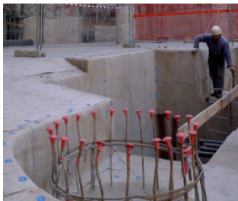
Waterproofing a top-down roof with Mapeproof
