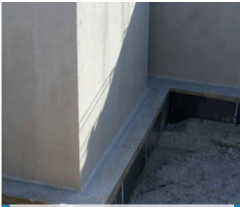
Waterproofing vertical surfaces with Mapelastic Foundation
