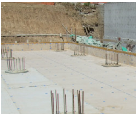
Waterproofing a foundation slab with through piling
