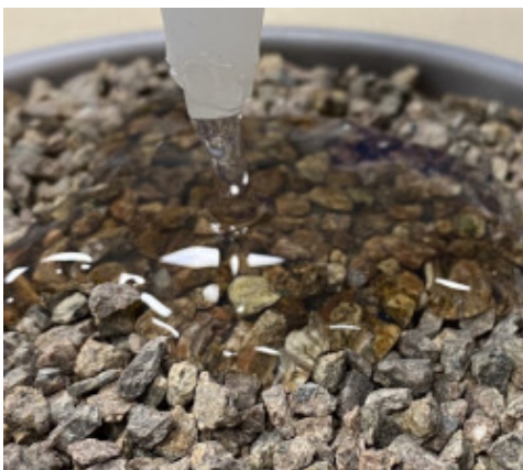
Application of Mapestone Joint Ghost
