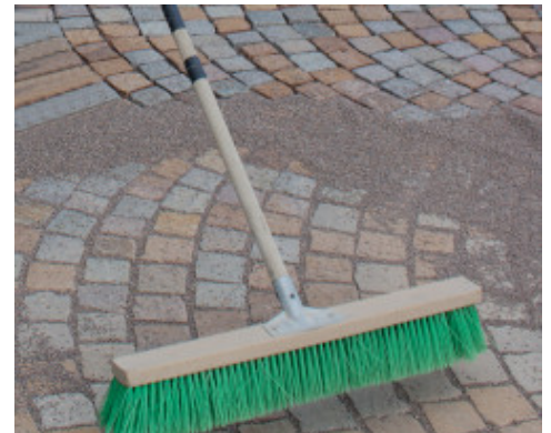
Filing the joints with fine gravel
