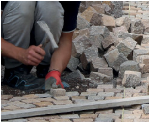
Placing the porphyry cobbles in position
