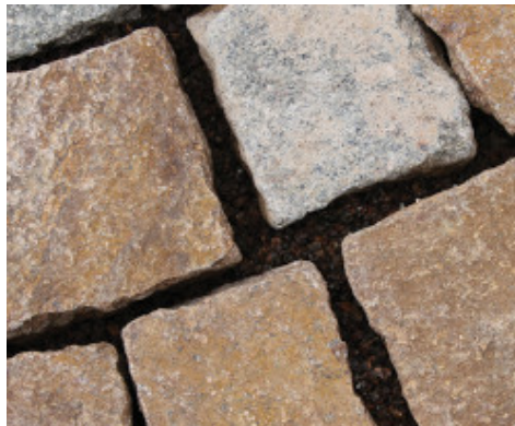
Close up of the newly-laid cobbles
