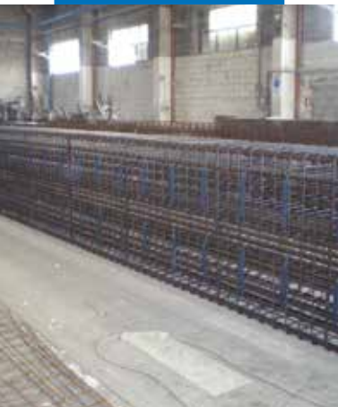
Mapeshield I welded to the reinforcement of a new beam in the construction of a dockyard quay
