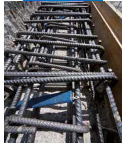
Construction of a new central reservation protected with Mapeshield I
